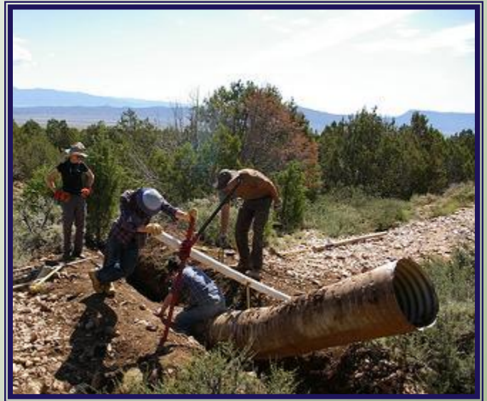
BTCV Crew Members Removing Culvert
